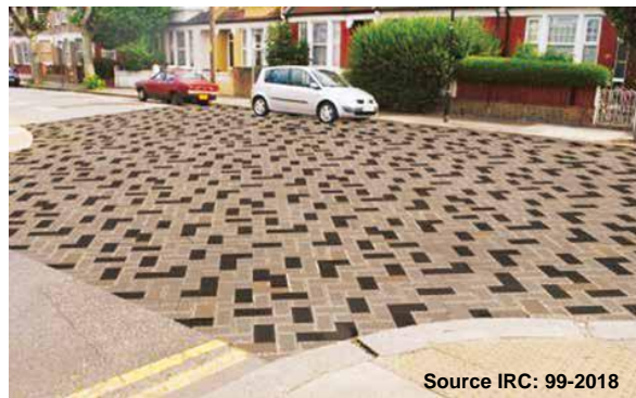
Figure 10 Textured Paving over Raised Crossings
